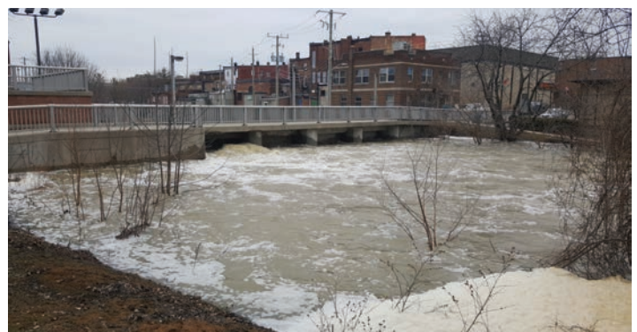
The 6th St. Backwater Dam and Pumping Station in Chatham continued operation on February 24, holding back the highest flows since construction in 1992.
