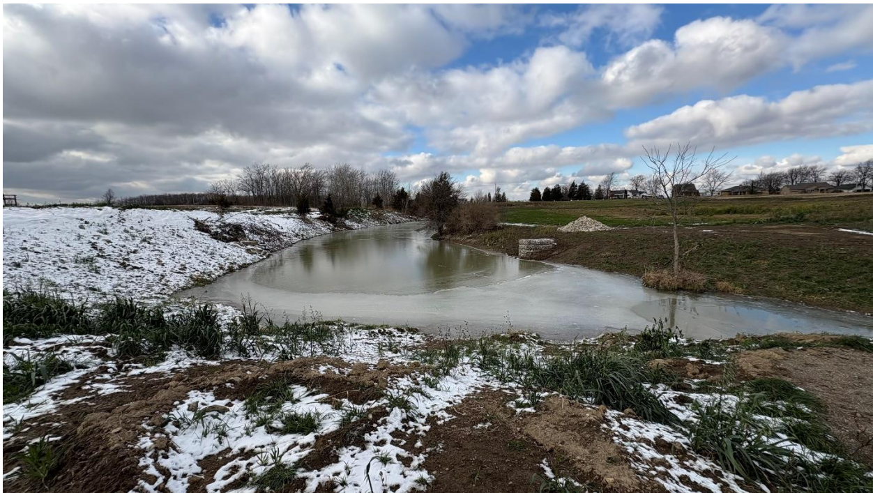
Checking up on a South Kent project in the Winter. The wetlands went into the cold season with a thick growth of oats to help with erosion, and the "fish crib" is working as intended.
