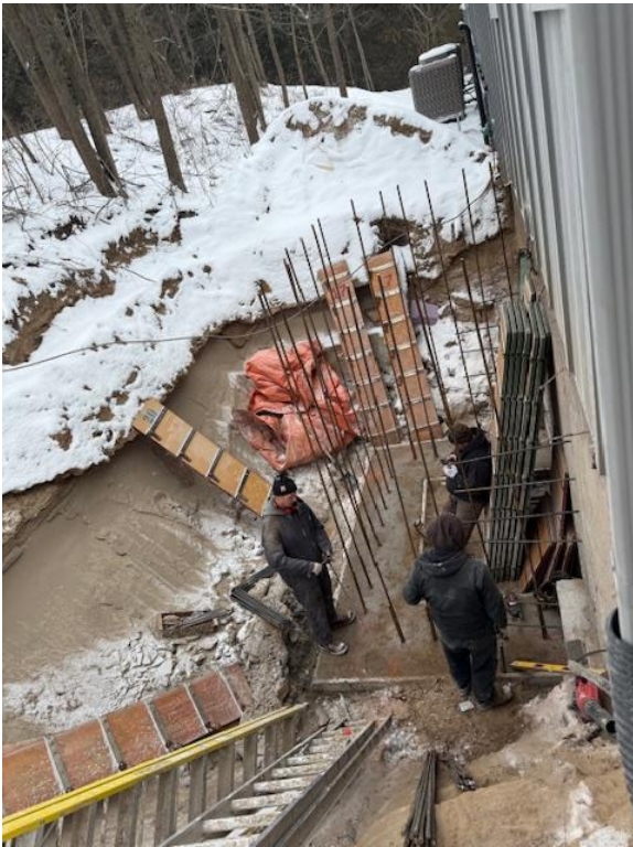
Elevator Construction at Longwoods Road CA.
