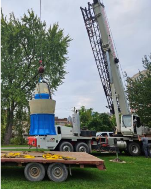
Photos: Pumps being reinstalled, and removed for servicing, October 1 st , 2024
