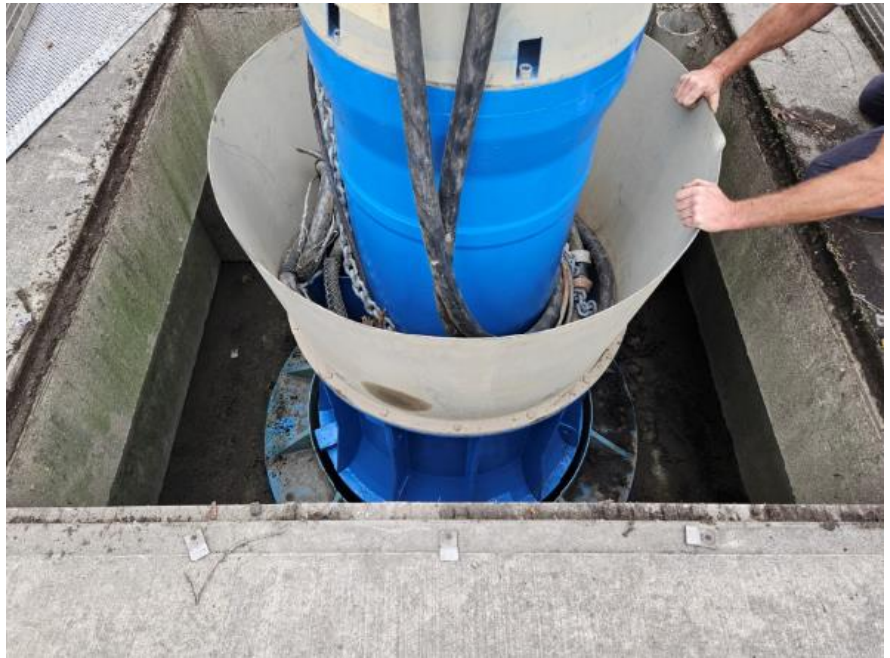
Photos: Pumps being reinstalled, and removed for servicing, October 1 st , 2024
