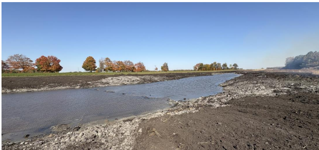
Completed 2-acre wetland in Muirkirk
