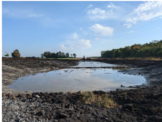
2-acre wetland in Muirkirk, under construction
