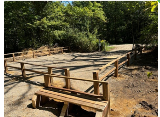
New parking lot at Mosa Forest Conservation Area
