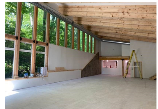
Inside view of the addition at Longwoods Road Conservation Area
