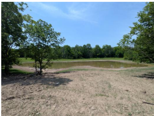
Wetland site (two weeks after construction) for project ID - LTVCA-01050H-C0343
