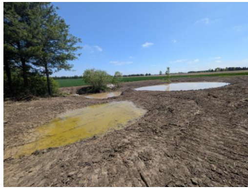
Wetland site (One week after construction) for Project ID: LTVCA-00625M-C0544
