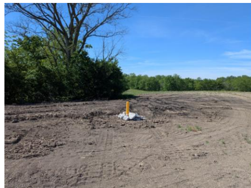
Looking at 1 WASCOB area for project ID - LTVCA-01050H-C0343
