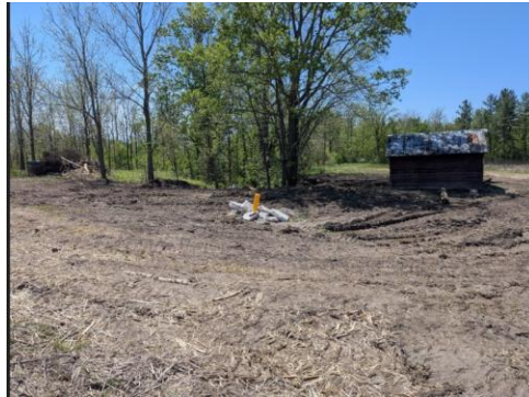
WASCOB Area for (Day after construction) for Project ID: LTVCA-00625M-C0544
