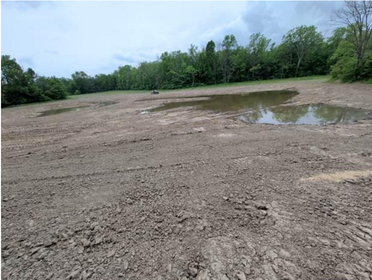
Completed Wetland at Geraldine Hind's Farm.
