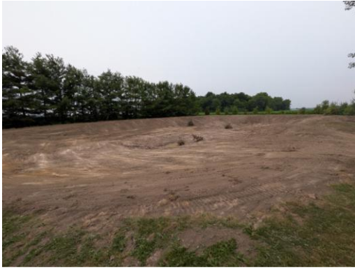
Wetland Site (Day after construction) for Project ID: LTVCA-00434H-C0707
