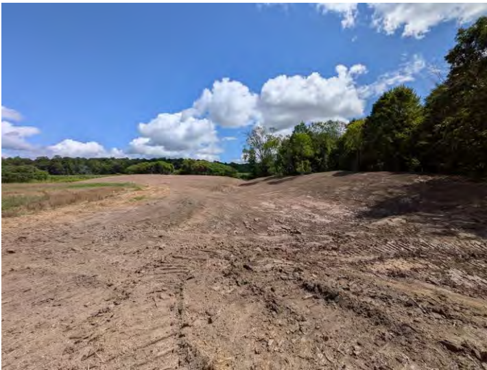
Wetland site (Day of completion) for project ID - LTVCA-01760S-C0762
