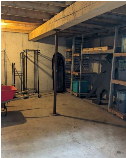
Oneida Cabin Basement
