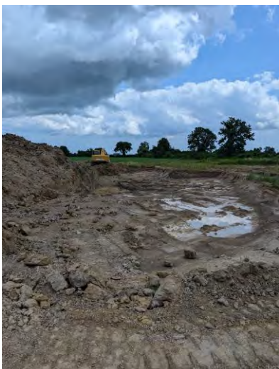
2024 Cedar Springs Wetland - Before
