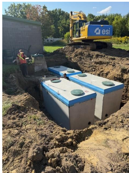
Photos of the Water System Tanks being installed.
