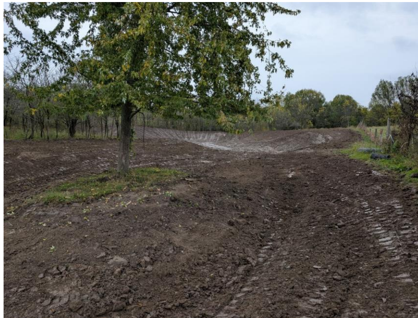
Gustin Wetland Site near West Lorne- 0.4 acres (day after construction)
