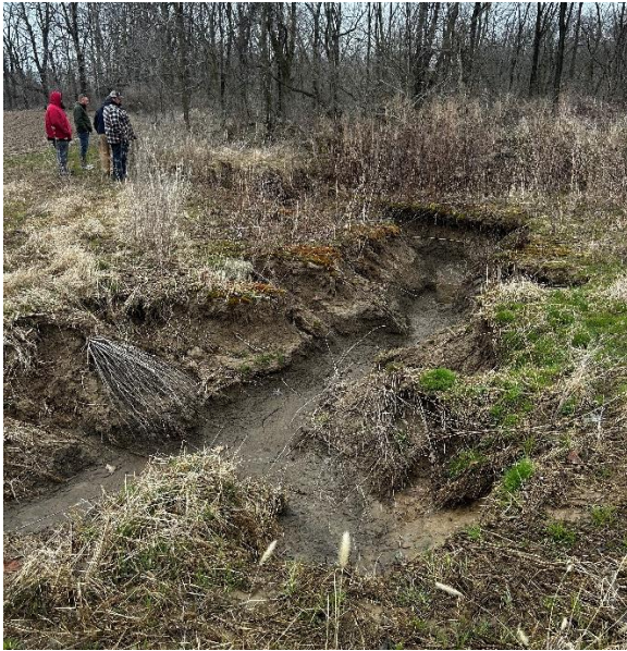
2025 Smith Erosion Control Project – Initial Site Visit
