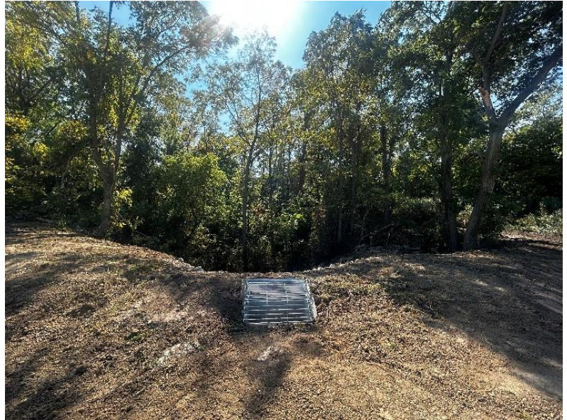
2025 Smith Erosion Control Project – Completed Construction
