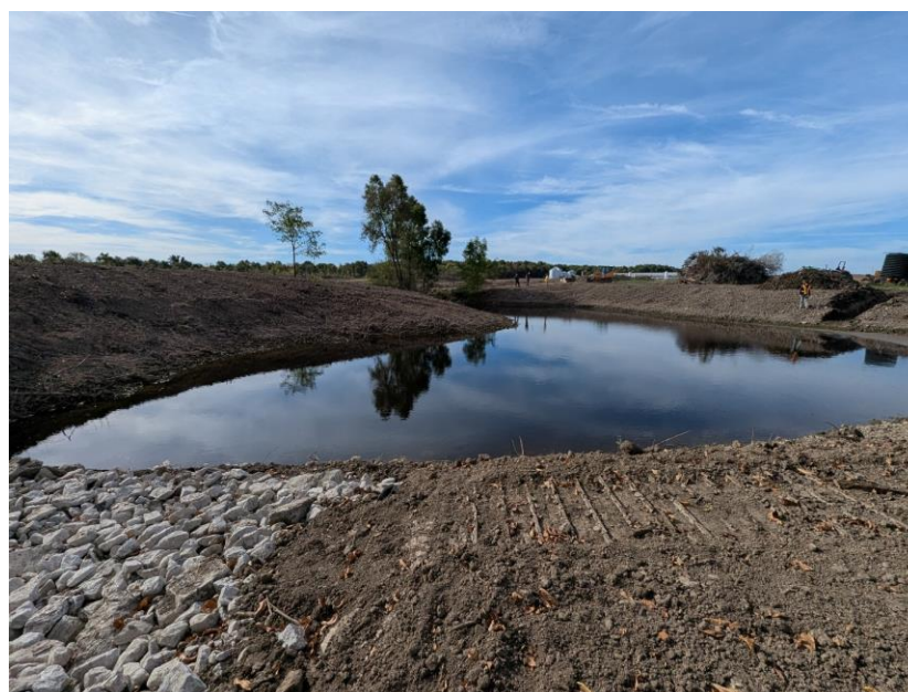
Buis Wetland & Erosion Control Site near Glencoe- 0.4acres (Few Days after construction)
