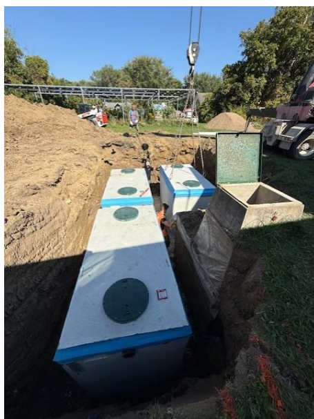
Photos of the Water System Tanks being installed.
